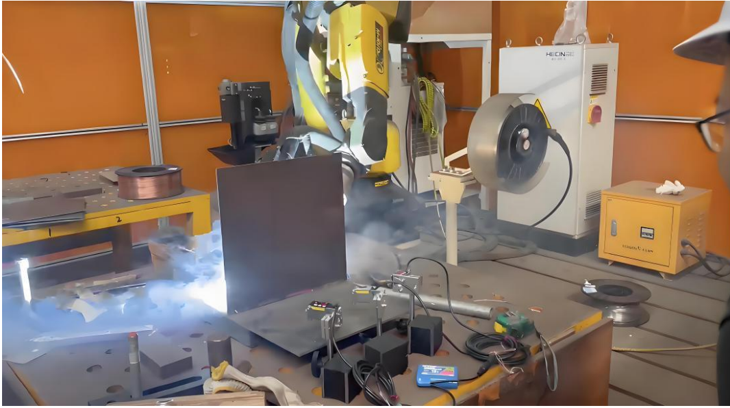
Figure 2 Field welding process
